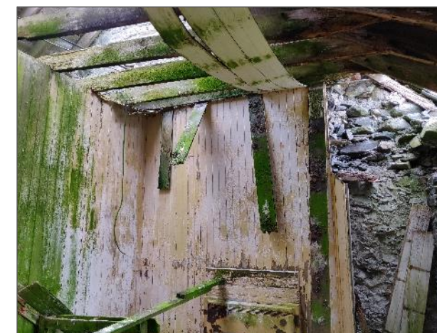
Photograph 6 Internal view of crofter's cottage showing collapsed roof
