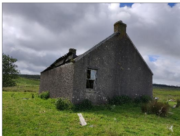
Photograph 4 Derelict crofter's cottage with concrete rendered walls
