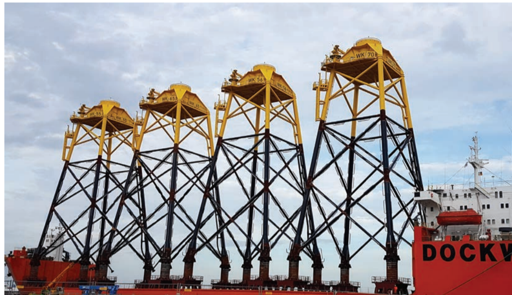
Main image: 65-metre-high jacket foundations ready to be installed at the Wiking windfarm site.
