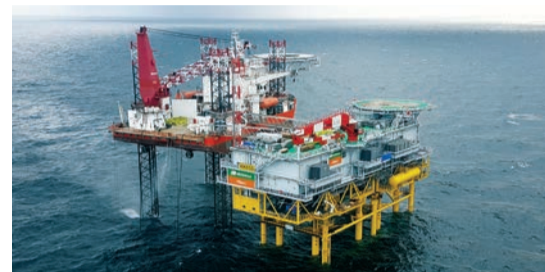
Wiking's offshore substation 'Andalucia' being installed in the Baltic Sea
