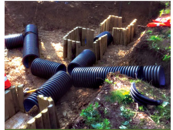
Above, bottom left: construction of the artificial badger setts
