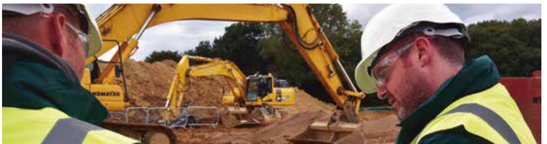
Construction underway at Bramford
