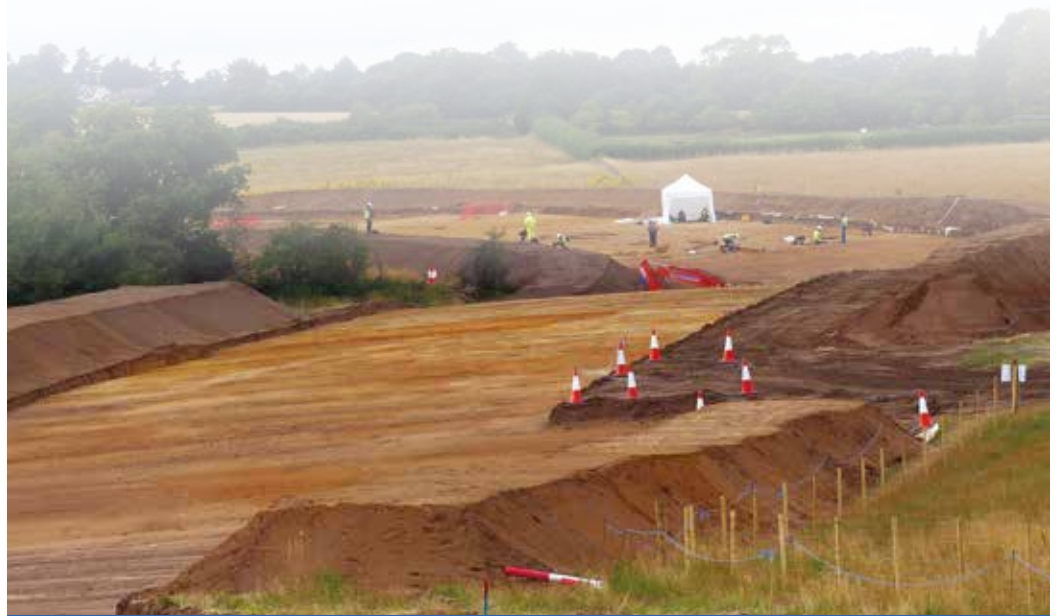
The top soil has been stripped to allow archaeological works to take place
