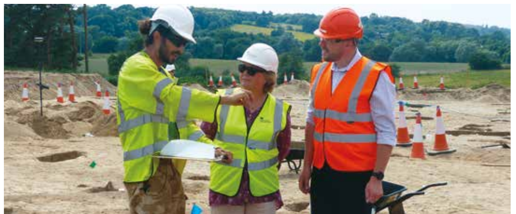
The Mayor of Woodbridge, Clare Perkins, visits a site to see the works
