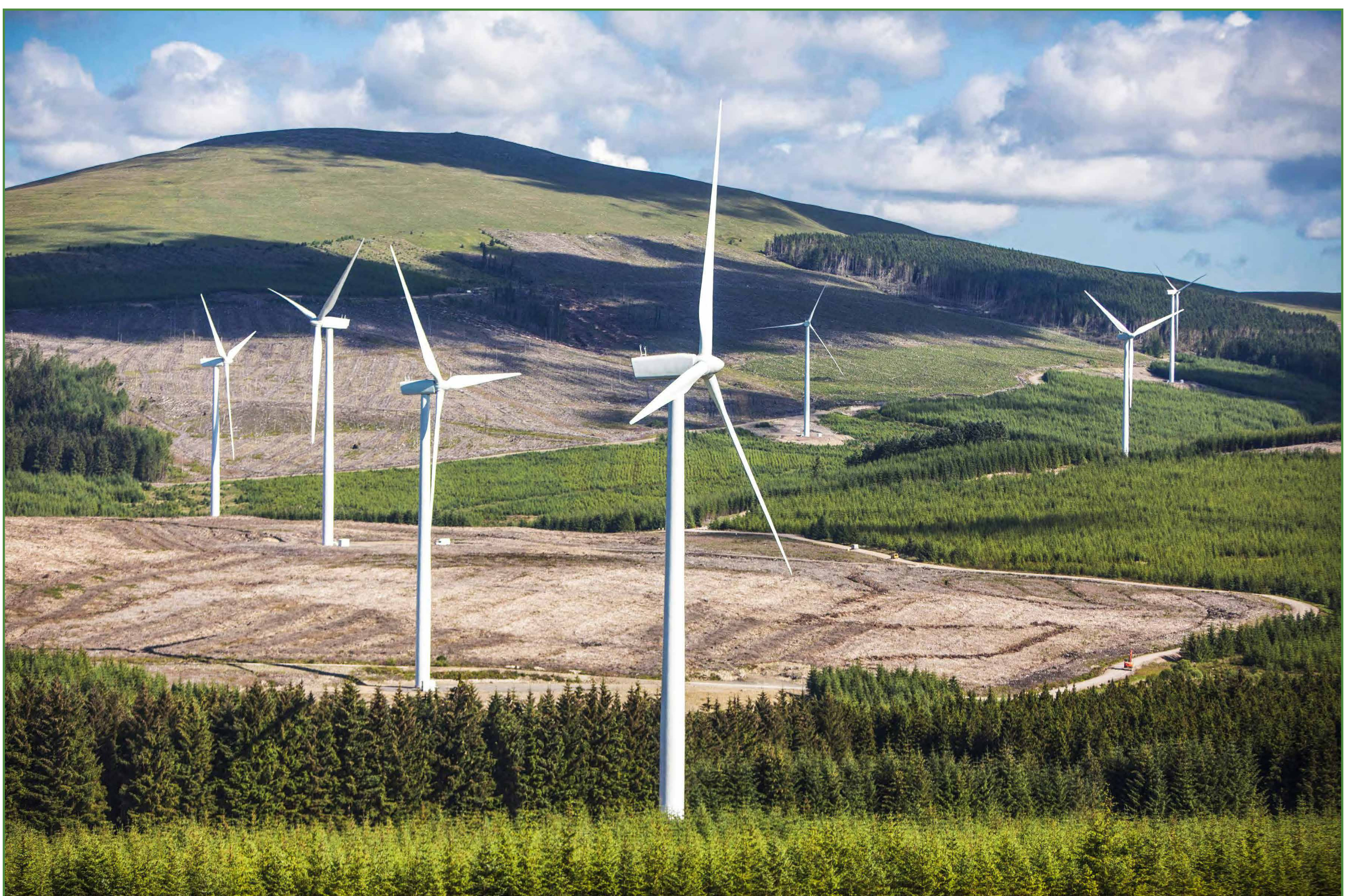
Harestanes Windfarm, turbine tip height up to 121.5m
