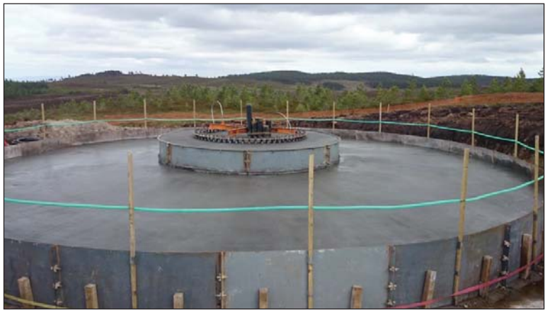
Plate 10: Typical wooden shuttering – to be deployed around the turbine foundations during concrete pours
