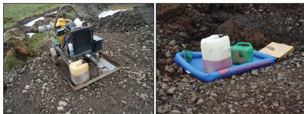
Plates 11 and 12: examples of drip trays and bunds
