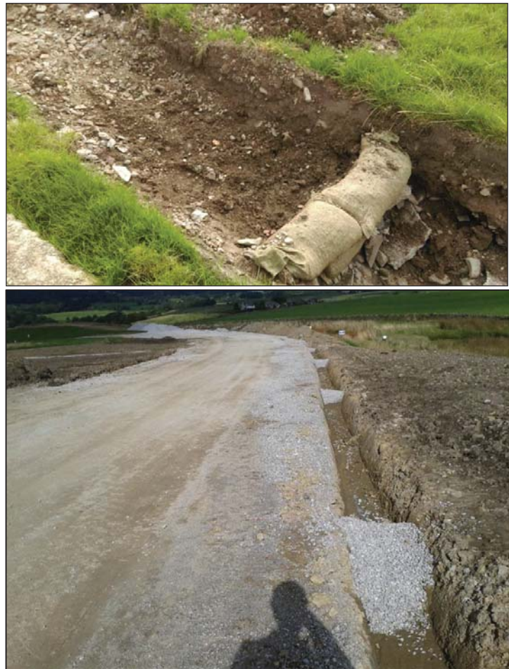
Plate 4: Typical check dams - to be installed in drainage ditches adjacent to the access track
