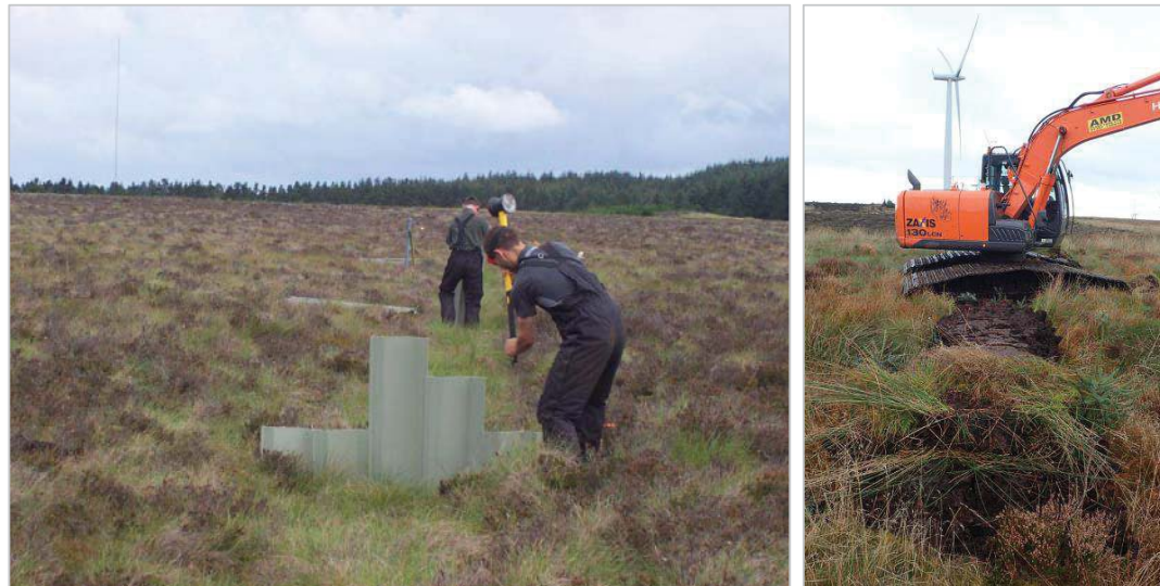
Photos 8 & 9: Plastic piling (left) and conventional peat dam mid construction (right)
