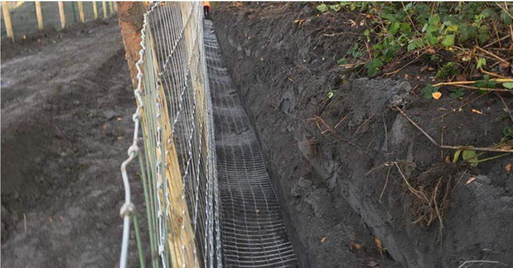
Figure 6.8 Installation of Badger Fencing
