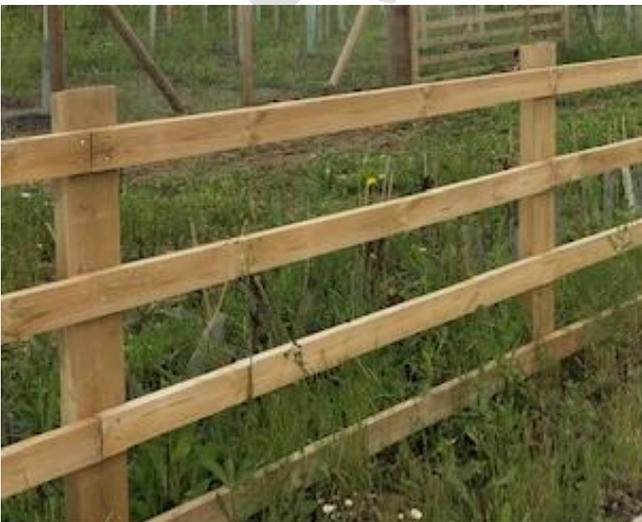
*Figure 6-2 Post and Rail Fencing*
