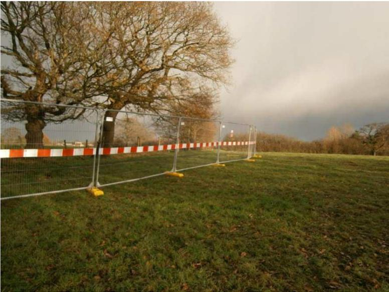
**Figure 6.6 Example Heras Fencing Tree Protection**
