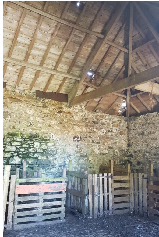
Figure TA_8.3.4 - Inside of stone barns
