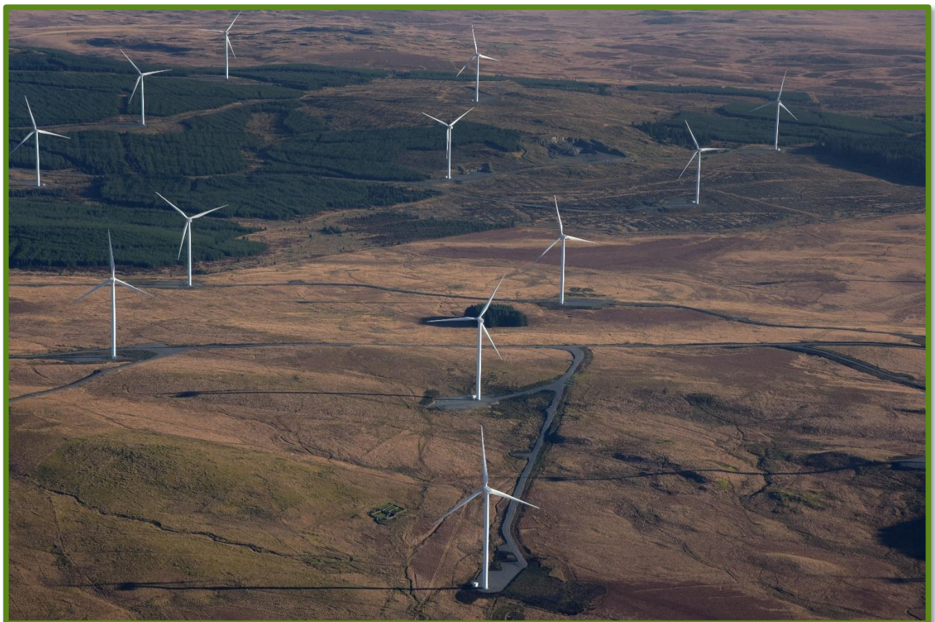
Figure 2 – The existing operational Kilgallioch Windfarm, which has turbines up to 145.5 m to tip
