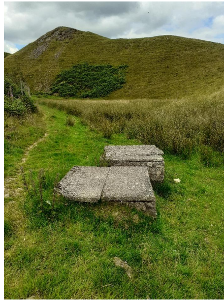
Photograph 6.4.1: PWS01 spring collector tanks at NGR 304597, 591656, looking north
