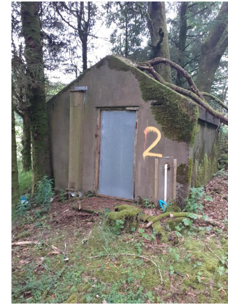
Photograph 6.4.3: PWS02, looking north towards the suspected supply source infrastructure at NGR 301197, 591131
