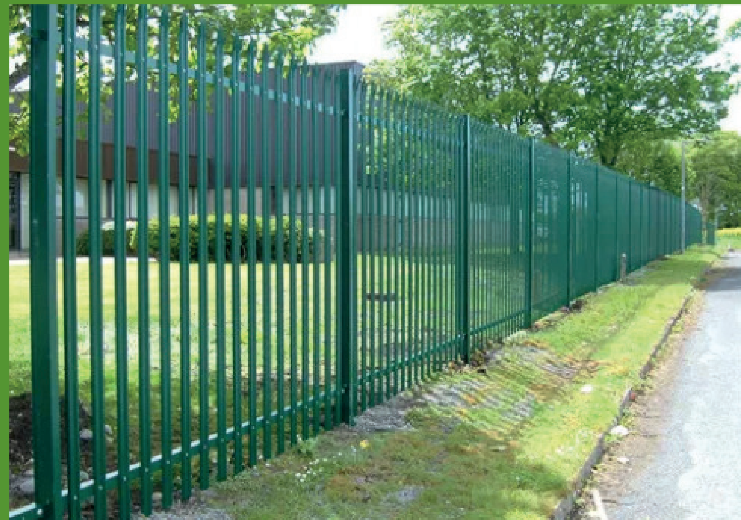
Typical Battery Storage Fence
