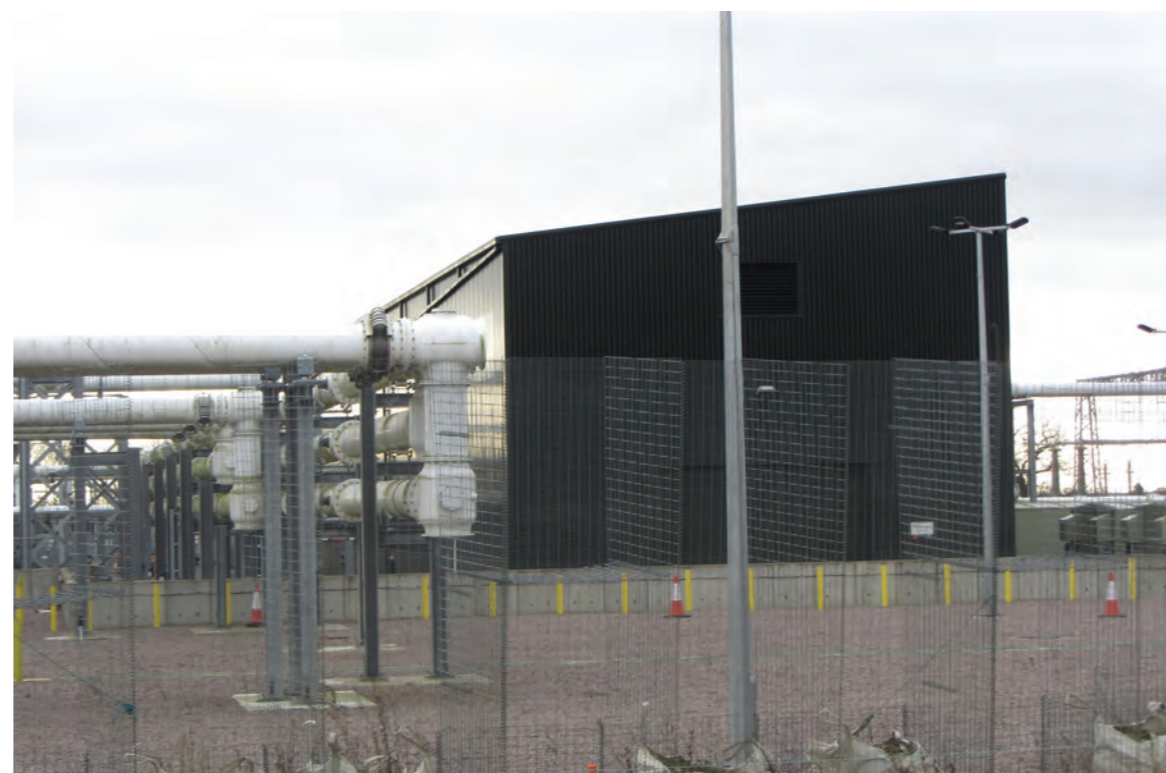
Bramford National Grid Substation
