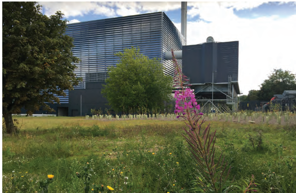
Great Blakenham Combined Heat and Power (CHP) Plant - an example of a high profile energy building
