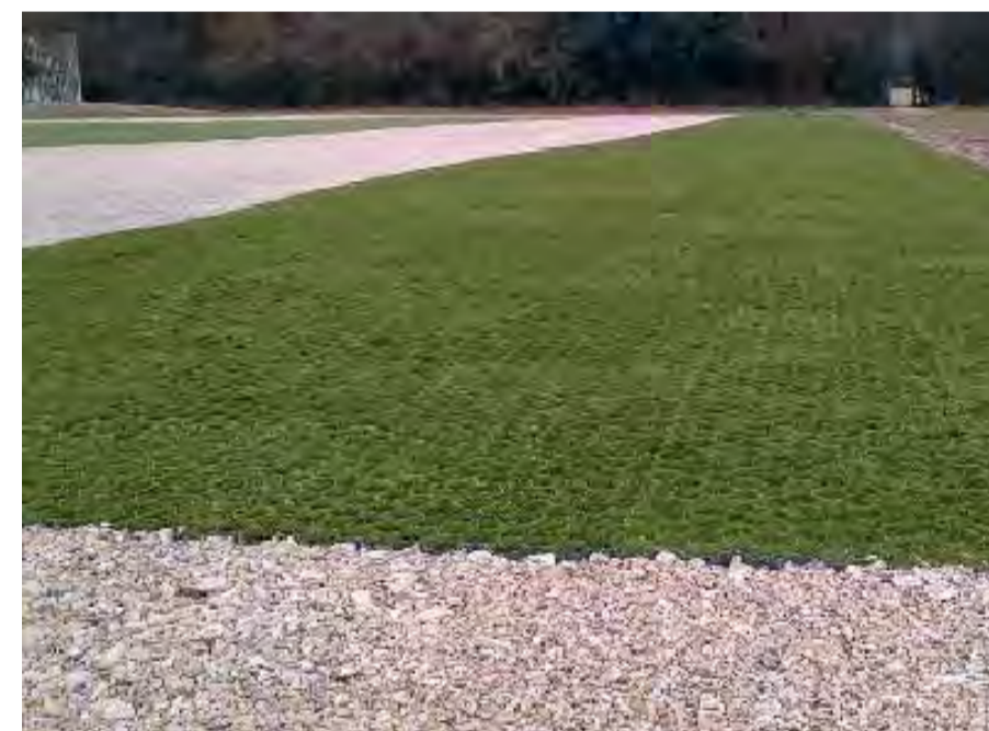
P4 - Installed grass road units
