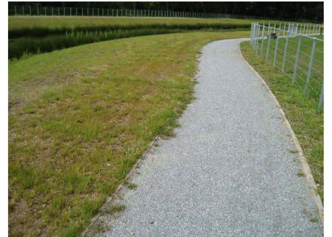
P3 - Installed self binding gravel path with timber edging
