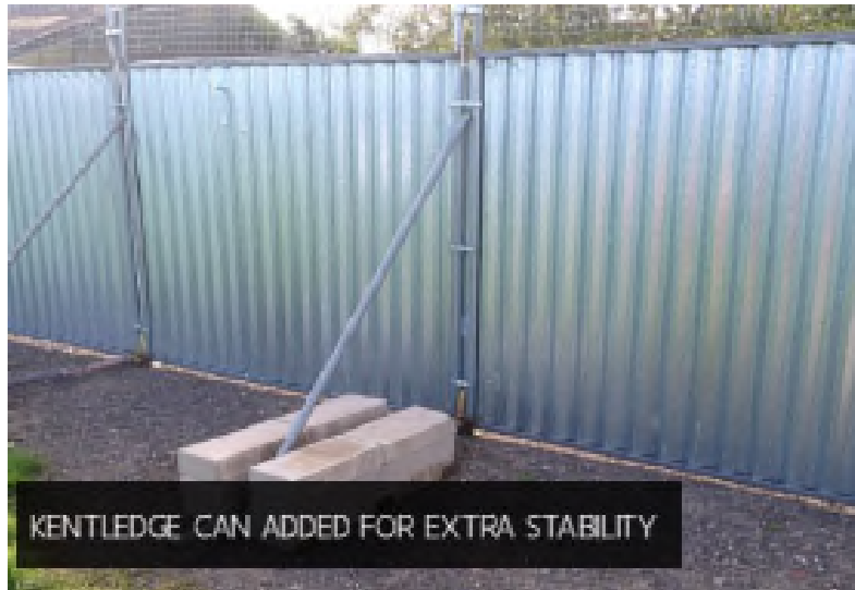
Figure 3.3 Example of Metal Hoarding Additional Support
