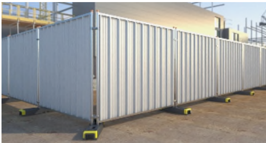
Figure 3.2 Example Metal Hoarding
