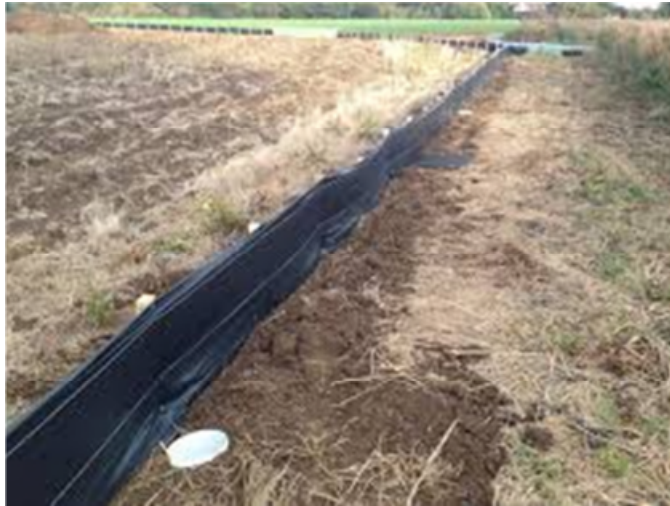
Figure 3.9 Example Temporary Reptile/Newt Exclusion Fencing
