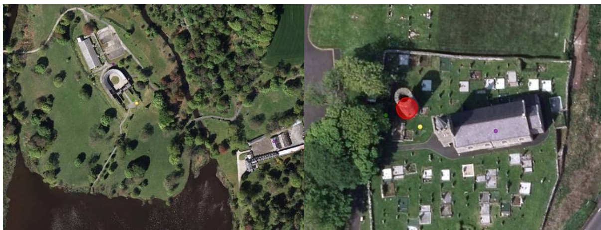
Plate 1: Snapshots provided by HED where yellow markers indicate visualisation locations with Lissanoure Castle on the left and Armyo round tower on the right
