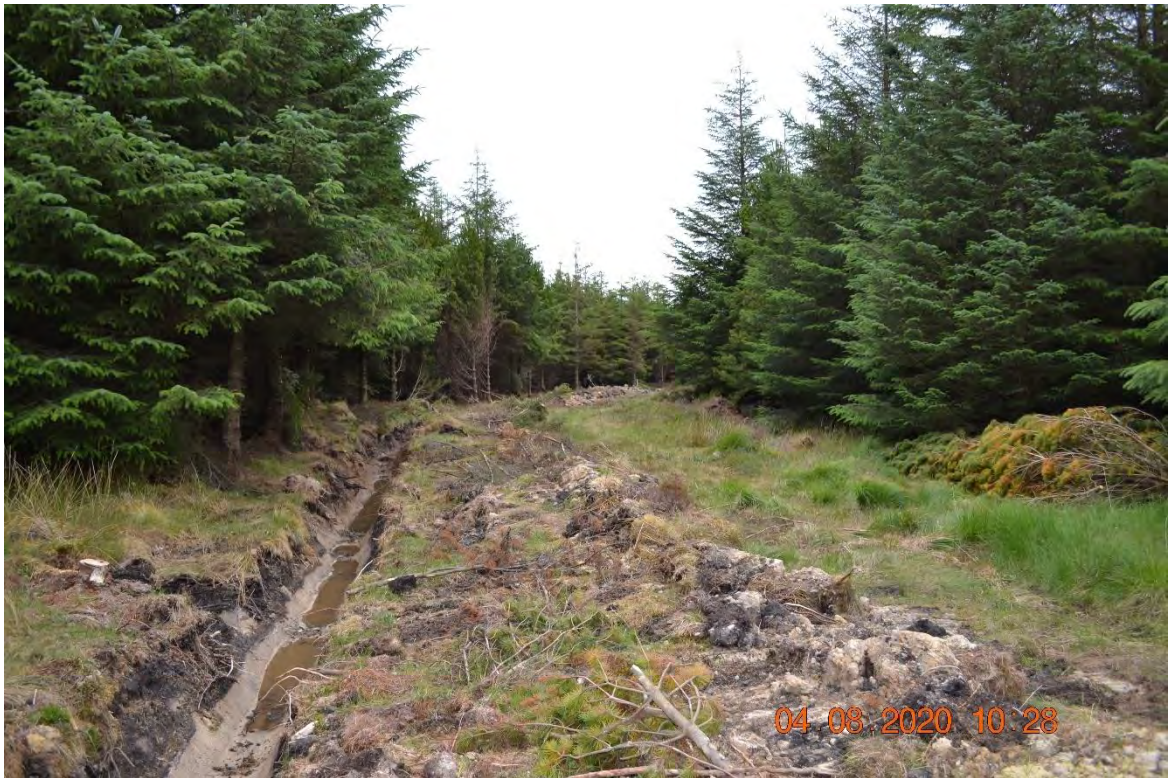
Figure 2: Turbine 1 location view to east
