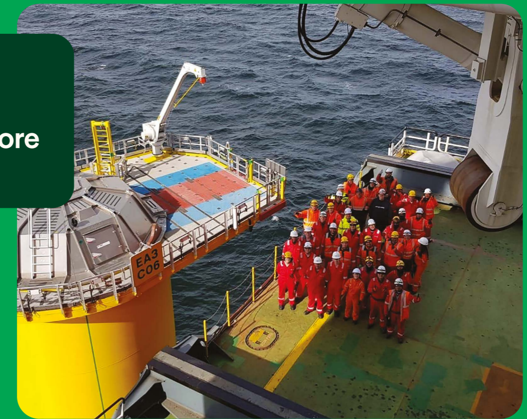
The SPR offshore team next to the first EA3 monopile, after the successful foundation installation
