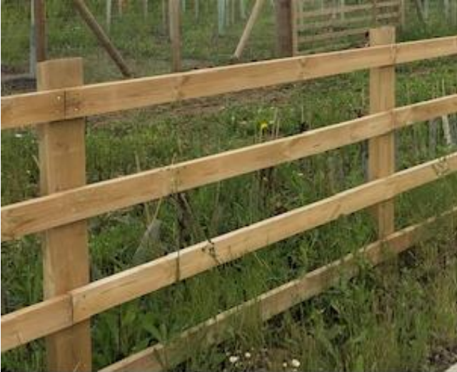
Figure 6.5 Post and Rail Fencing
