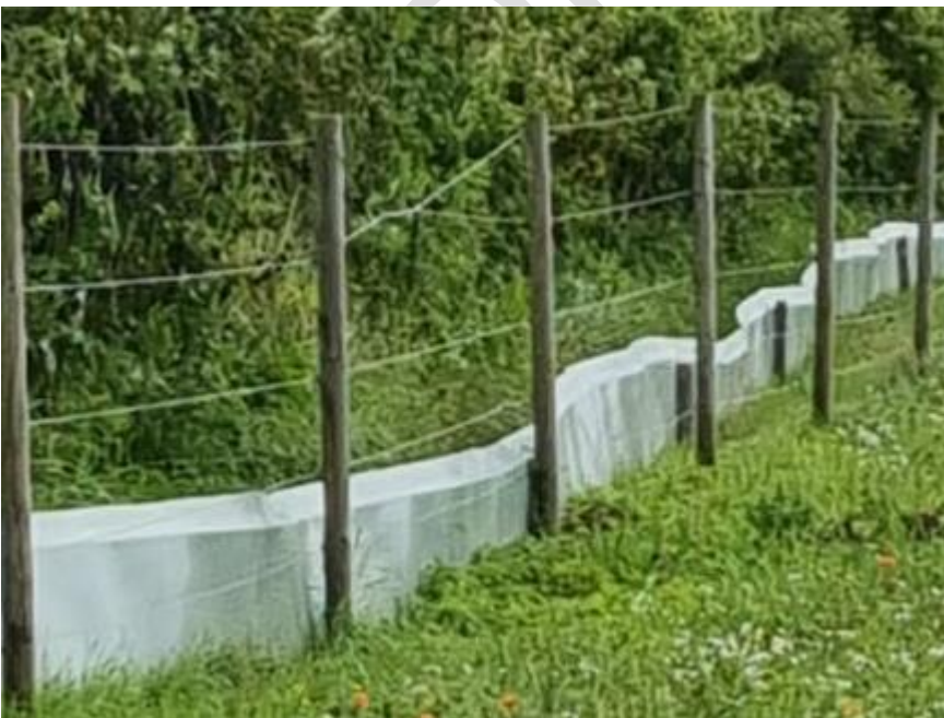
Figure 6-4 Post and Wire Fencing (with newt fencing behind)
