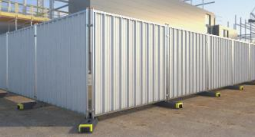
Figure 6-1 Example Metal Hoarding
