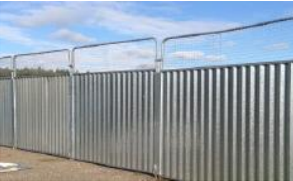
Figure 6-3 Example Extension Panels
