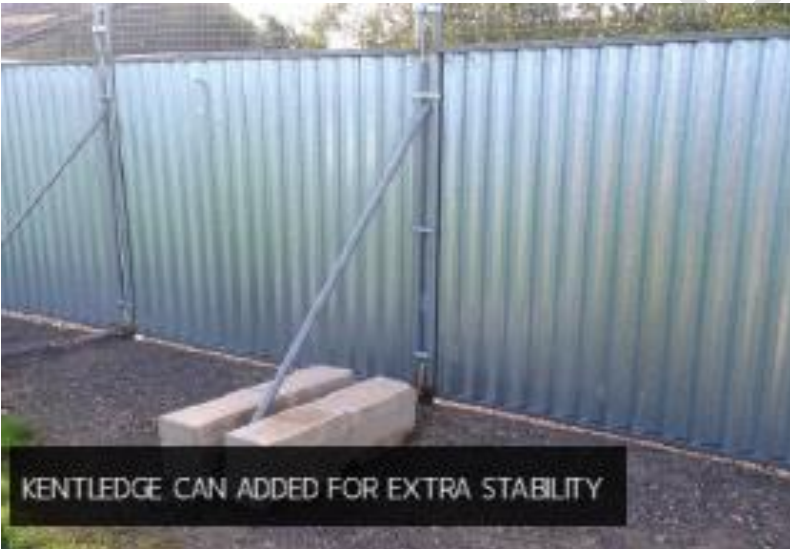
Figure 6-2 Example of Metal Hoarding Additional Support
