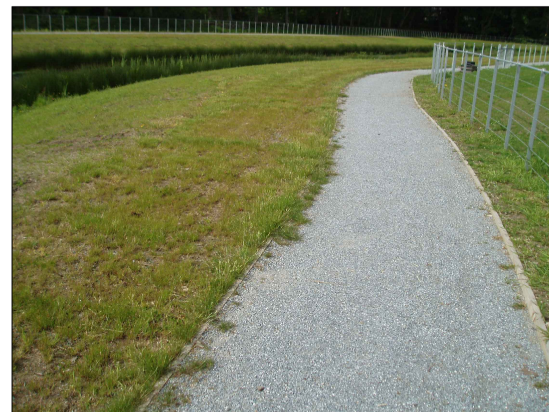
P3 - Installed self binding gravel path with timber edging
