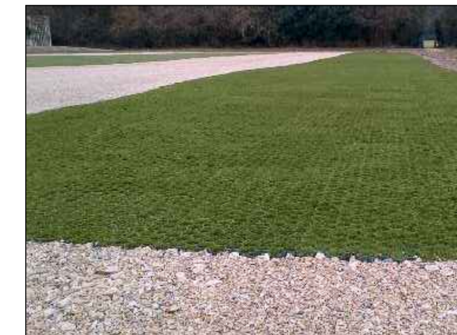
P4 - Installed grass road units
