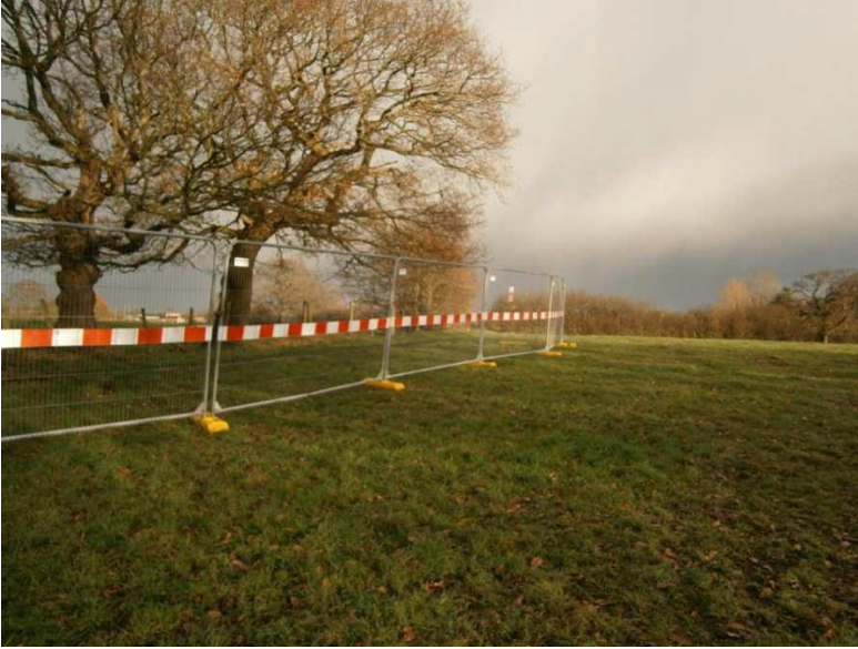
Figure 5.10 Example Heras Fencing Tree Protection
