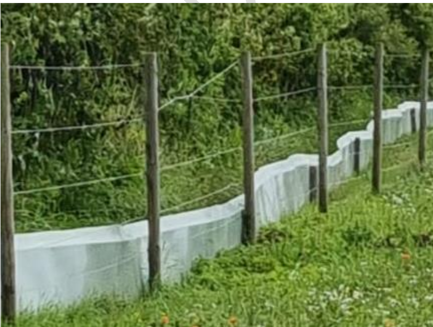
Figure 5.4 Example Post and Wire Fencing (with newt fencing behind)
