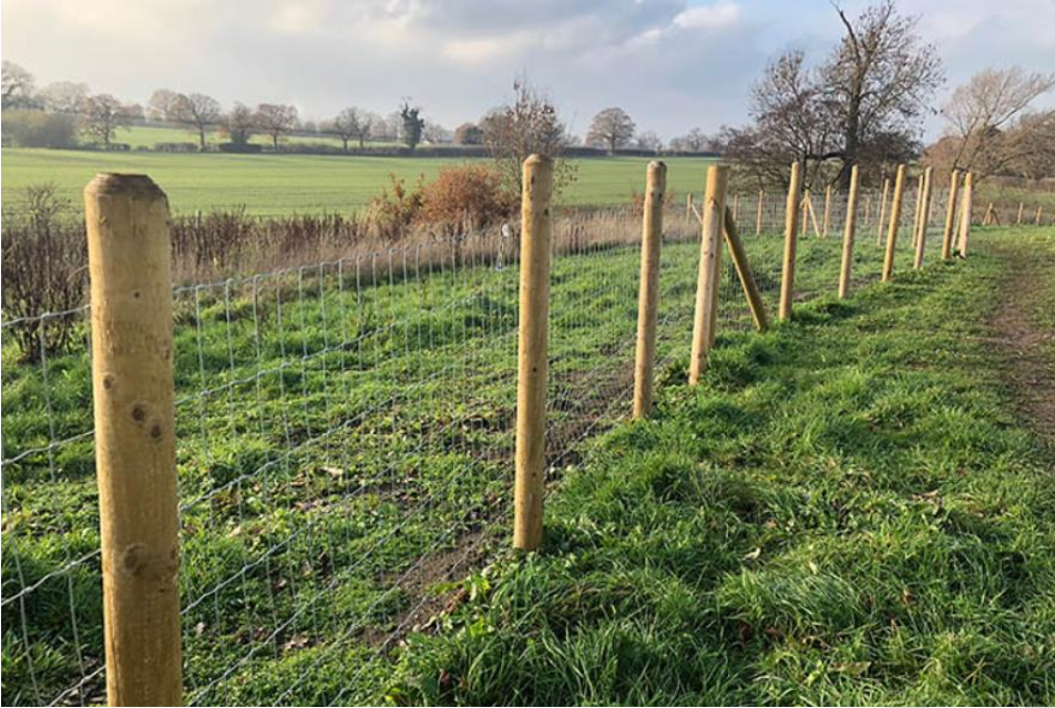
Figure 6.7 Example Badger Fencing
