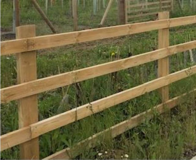
Figure 6-2 Post and Rail Fencing
