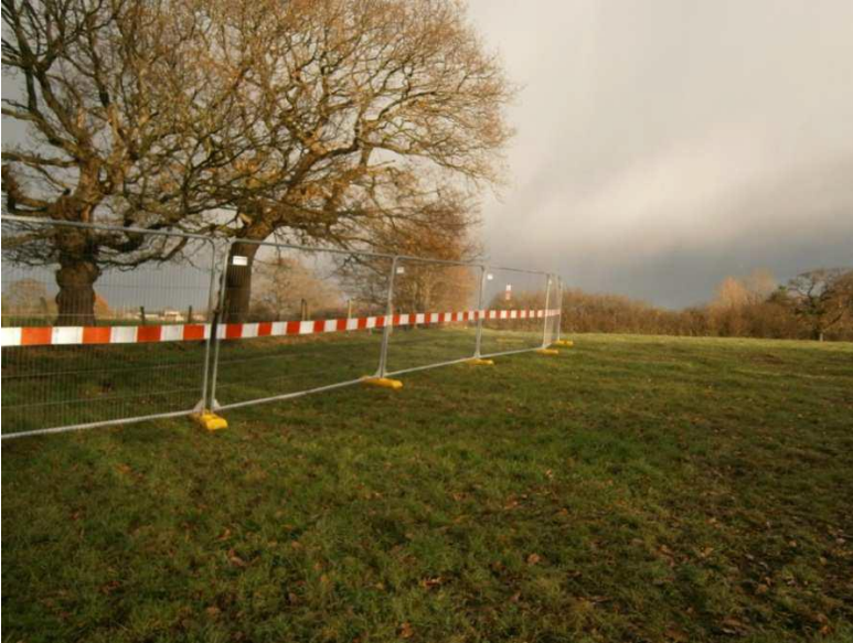
Figure 6.6 Example Heras Fencing Tree Protection
