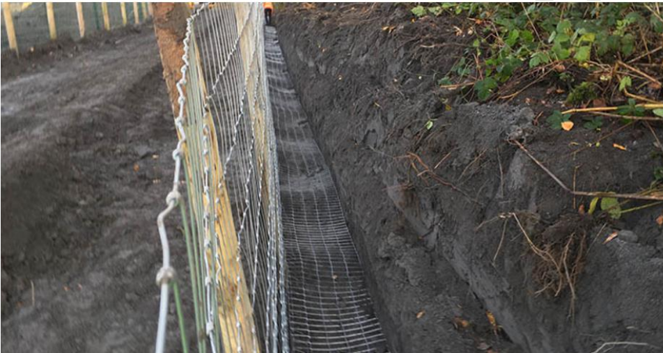
Figure 6.8 Installation of Badger Fencing
