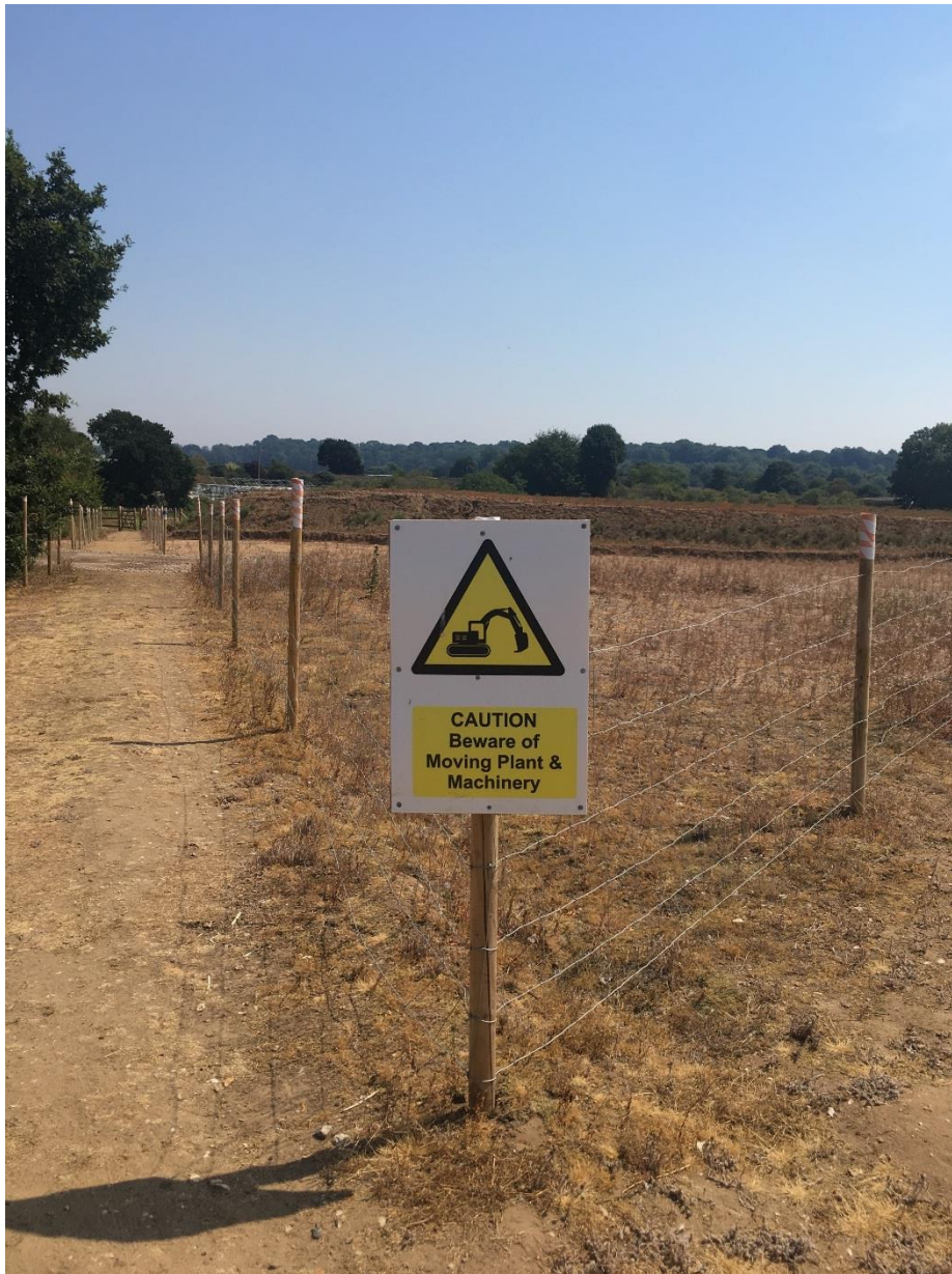
Plate 2.6 Example of a temporary fence used to delineate the boundary of the cable route working width (image taken from East Anglia ONE project)
