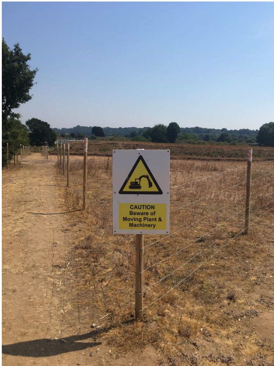
Plate 6.13 Example of a temporary fence used to delineate the boundary of the cable route working width (image taken from East Anglia ONE project)
